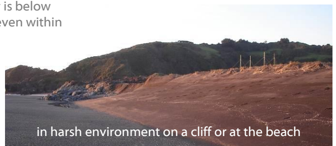
Active monopole antennas
